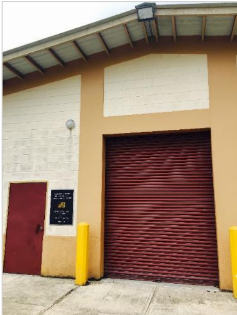
Figure 23. The Bluefields EOC and Central Warehouse, funded by USSOUTHCOM.
