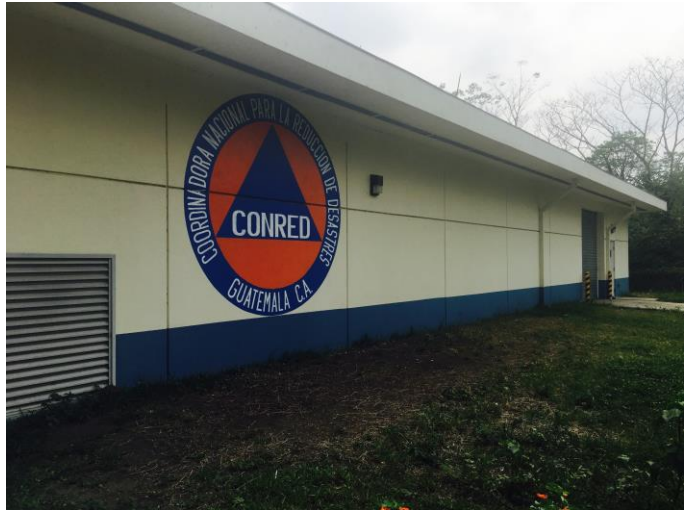
Figure 23. Escuintla Department (CODRED) EOC, offices, and warehouse
